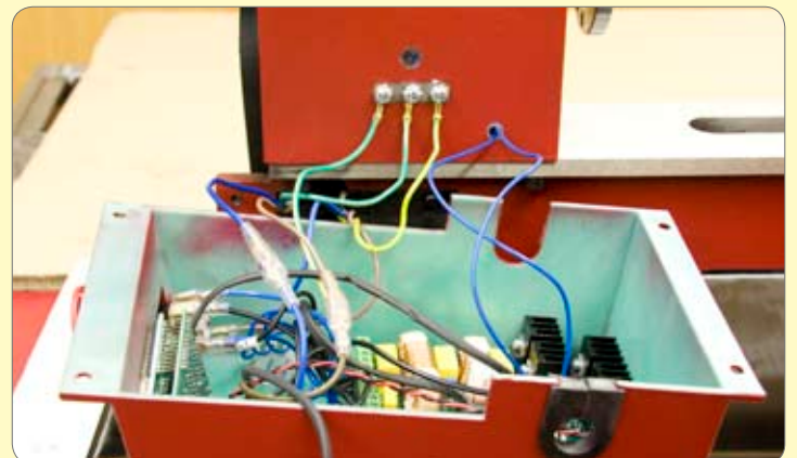
78. Reconnect all the wires to the control box.
